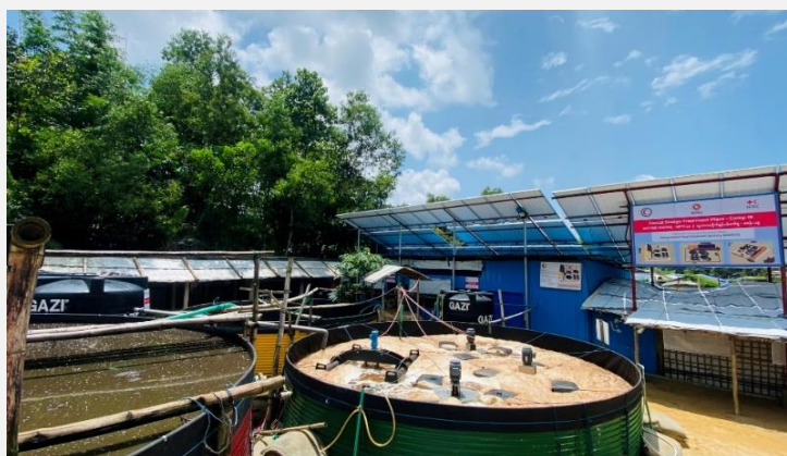
Households at D block of Camp 19 are benefited from this Faecal Sludge Management (FSM) plant (Photo: IFRC)
